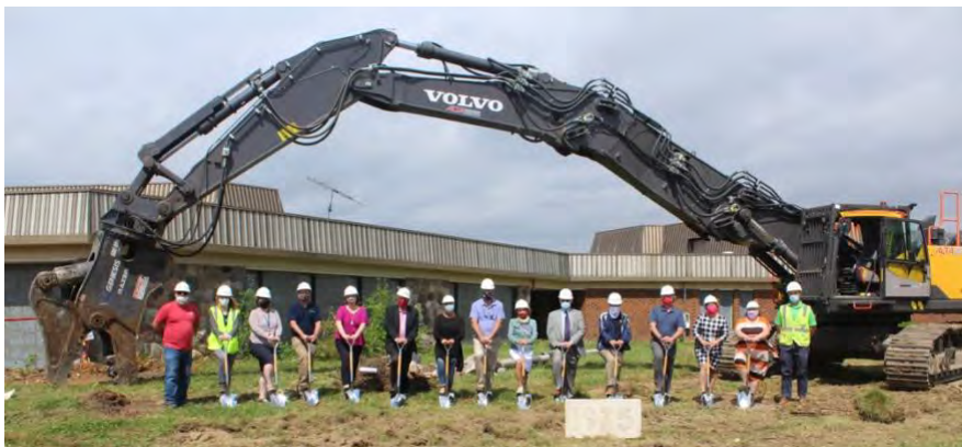
Pictured left: WISD administration, the Board of Education, and the design and construction management team pose for a groundbreaking photo.
